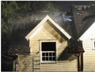
Fire official: Lightning sparked Cos Cob fire
